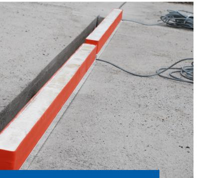
The Strain Gauge HS-WIM keeps costs lower than competitors by being durably built to last.
