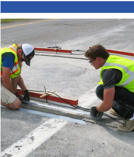
Installation is simple, flush-mounting the Strip Sensors into shallow cuts, reducing costs and operational disruptions.
